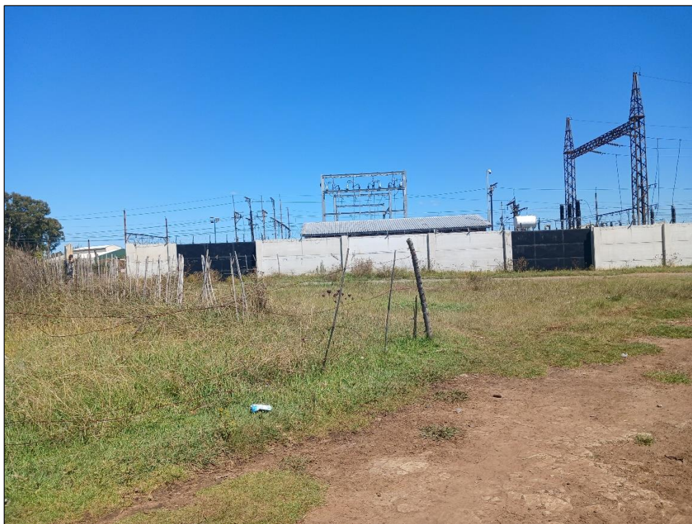
Figure 5: View of the railway substation.
